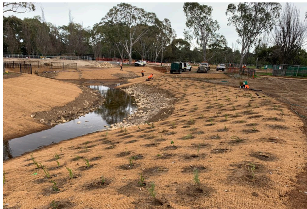
Park 20 - Planting commencing around the new open channels
